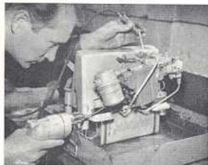
Fig. 1—Bench testing—fuel injection.
